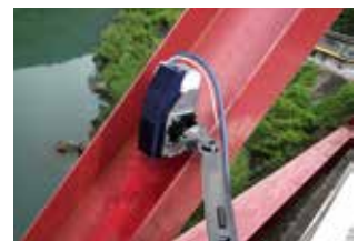
Bridges: Monitoring aging effects
